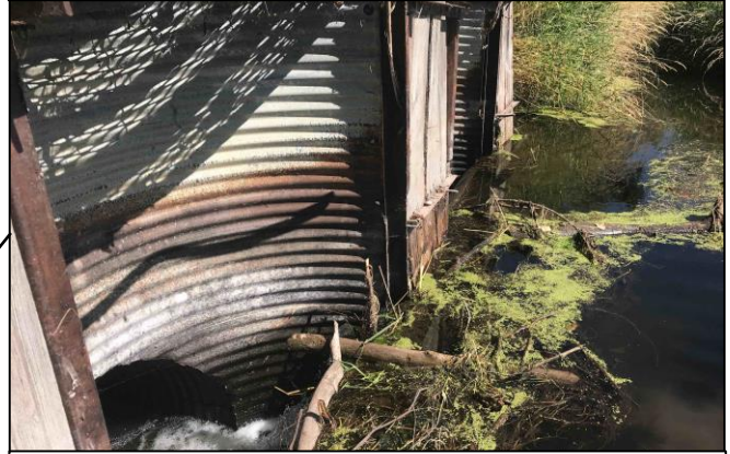
Relic check dam posing a fish passage barrier and altering natural streamflow and sediment mobilization.
