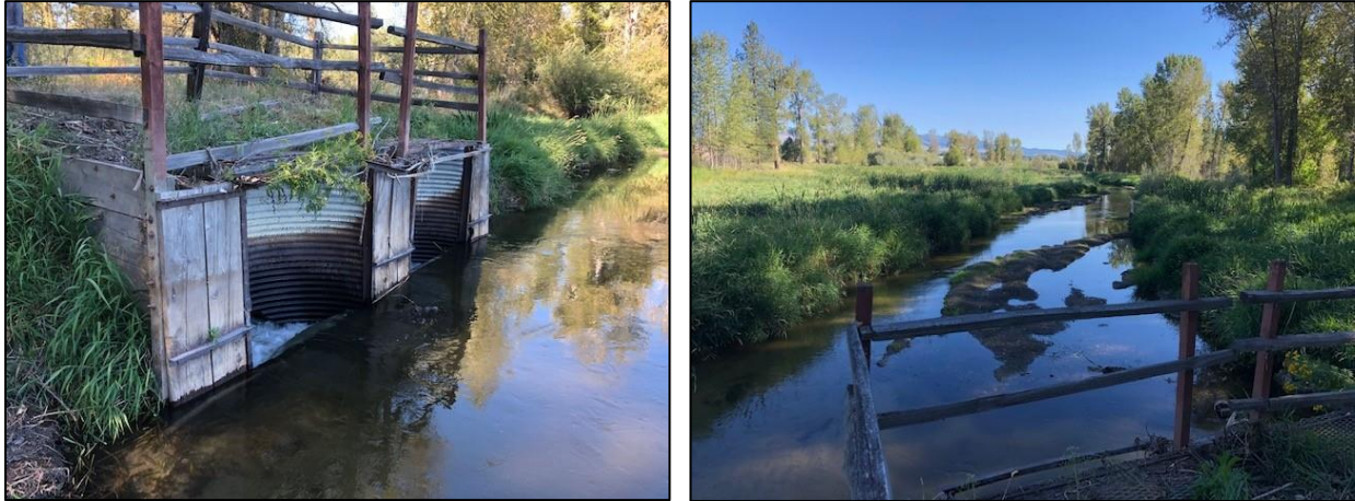
Figure 1-2. The existing relic check dam structure (left) and view upstream showing deposition of fine sediments, altered channel geometry, and impaired aquatic and riparian habitat conditions (right).
