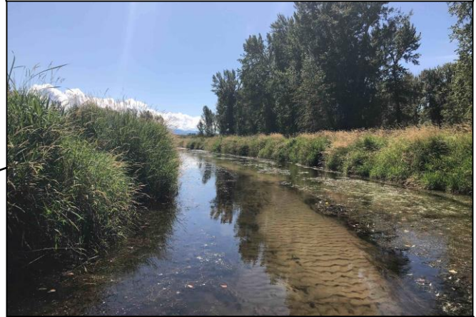
Sediment accumulated above the check dam structure. Reed canary grass comprises the vegetated cover.
