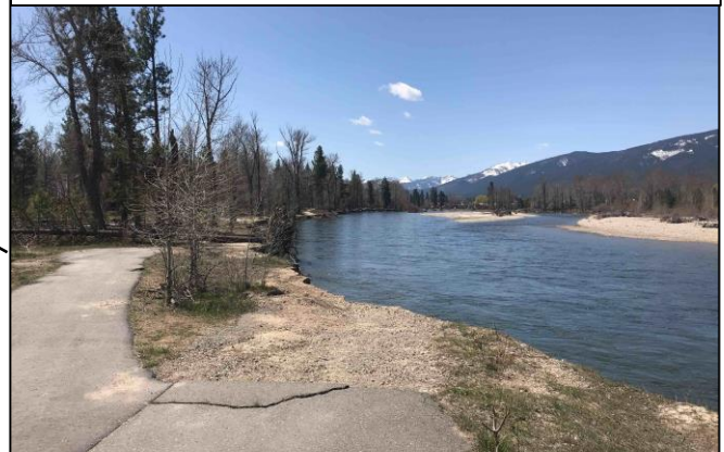
Natural channel erosion along the Bitterroot River. The river is expected to migrate to the current North Burnt Fork Channel in apx. 17 years.
