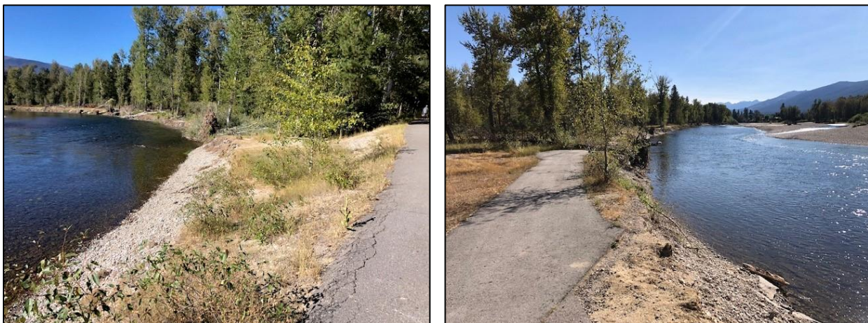
Figure 1-3. View of accelerated river bend migration and erosion, compromising the flood levee and walking path on the Refuge.
